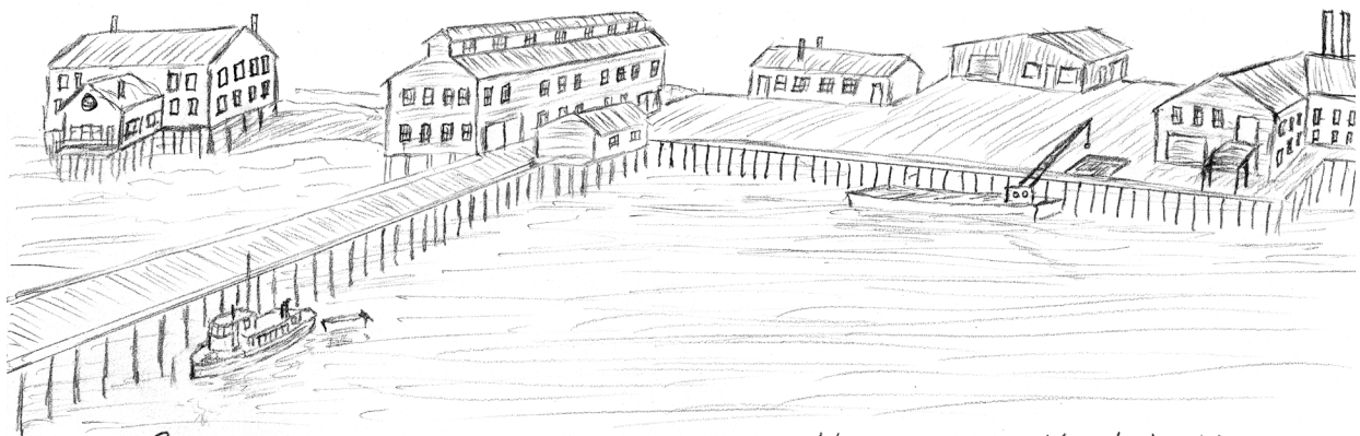
Pacific Endeavor Seafoods, August 1963. Buildings left to right: the bunkhouse with Sandy Ann's round window, the long net/can labeling/casing building, the little oil shed with Sandy Ann's thought spot, the mess hall, the store/warehouse, and the main cannery building with processing, retorts, boilers, and generators. The "Evangel" is at the long dock, and a barge and crane are working on the front dock.
